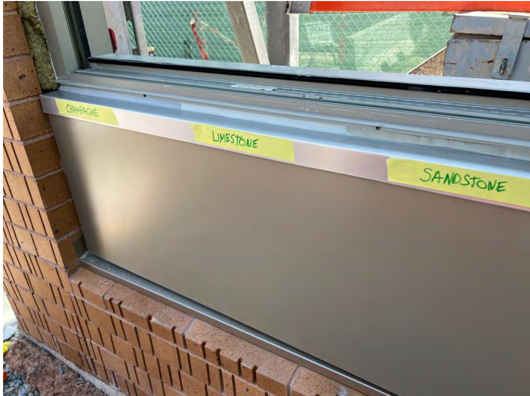
continued progress on the Mock up
