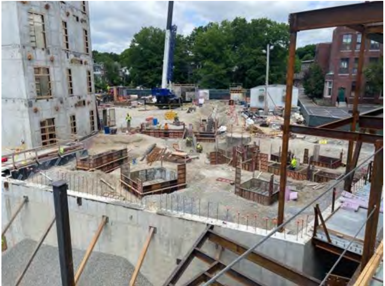
Rebar and forms at area ABC.
