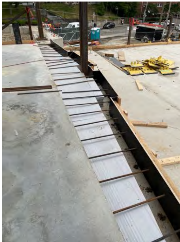
Deck 2C: forms, rebar, insulation.
