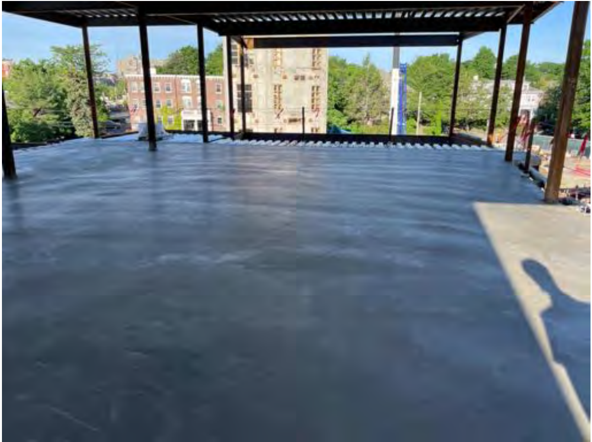
Finished slab at Level 3.
