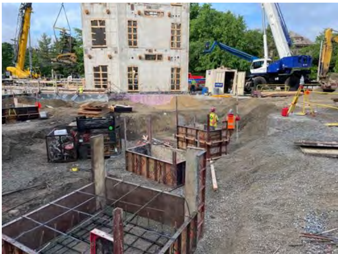
Excavation for forms adjacent to line A1.
