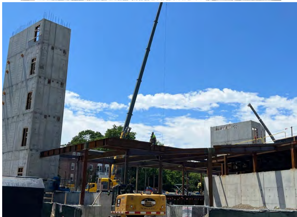
Steel&Decking Progress: view from the alley looking towards loading dock
