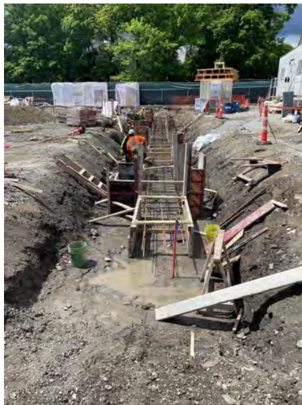
Footings at line BQ.
