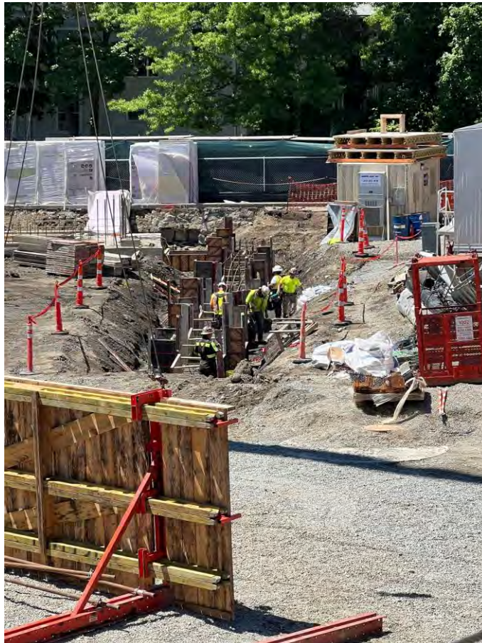
Forms and Rebar beginning on foundation walls at line BQ.
