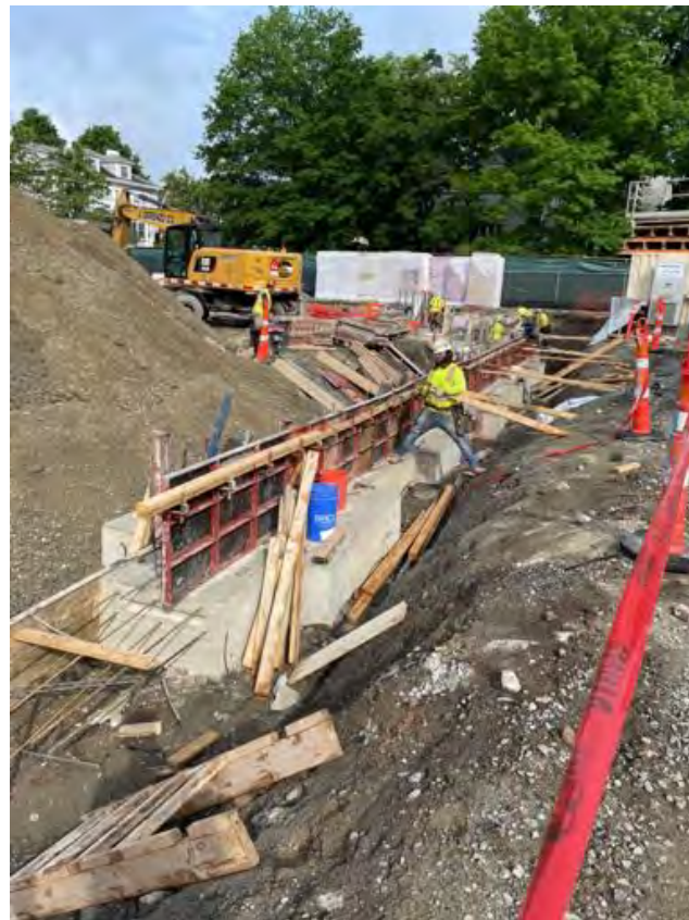
Line BQ wall forms.
