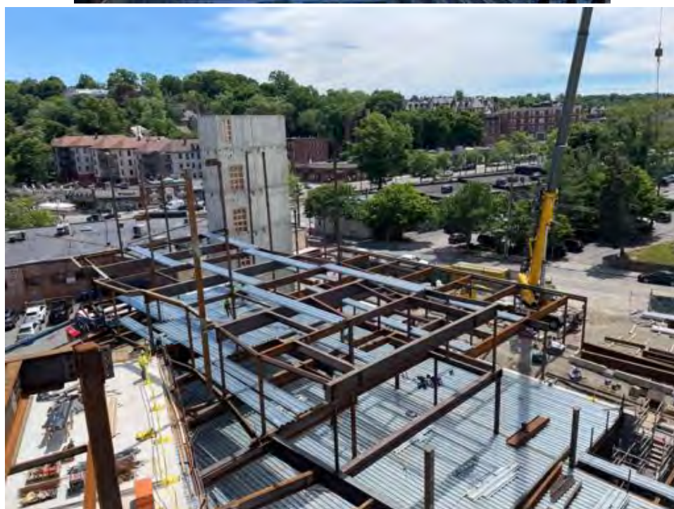
Steel erection, Area A.
