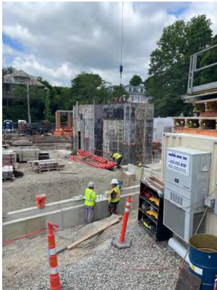
Starter forms at Core B.
