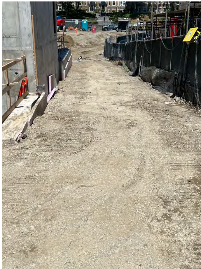
SOE removed, backfill and compaction completed along Alleyway
