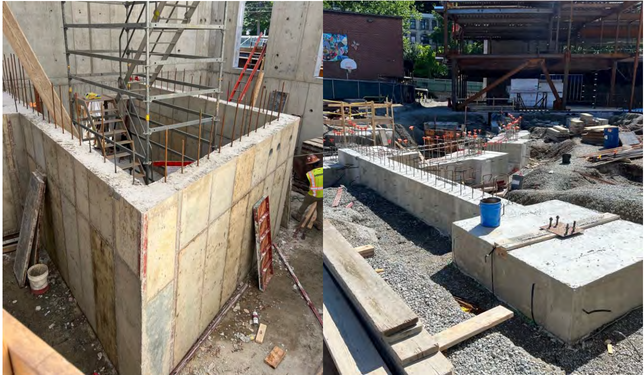
Forms removed from Friday's concrete pour.
