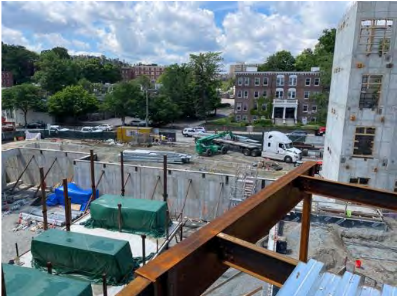
Delivery of deck for Building A.
