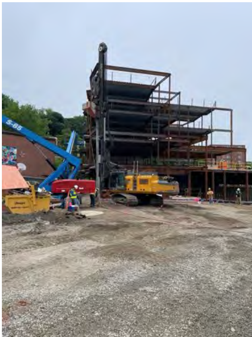
Geopiers adjacent to line A1
