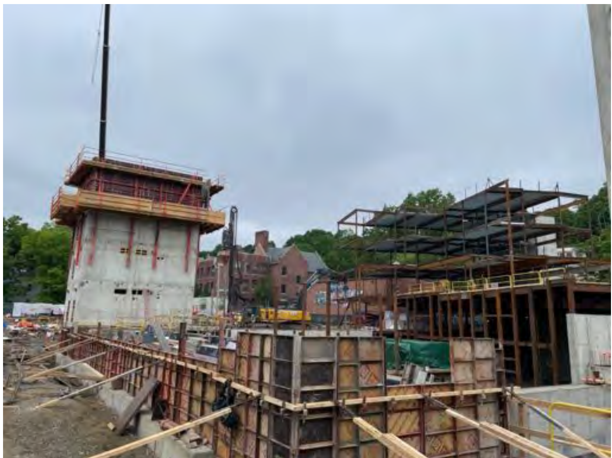
Stripped footings, installing wall forms – line AD.
