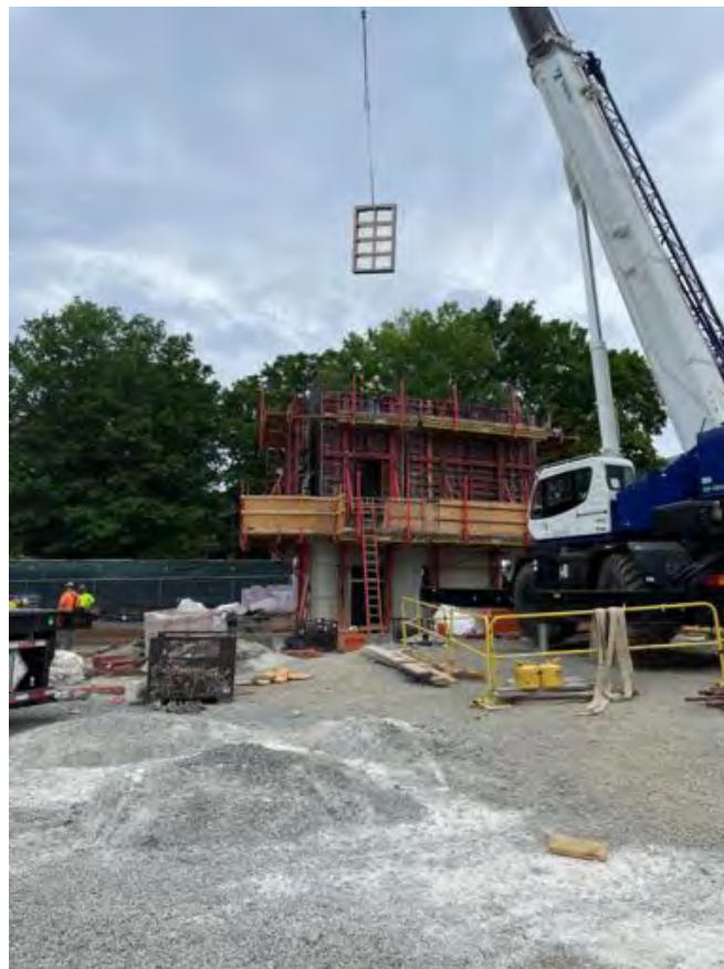
Core B rebar and forms ongoing.
