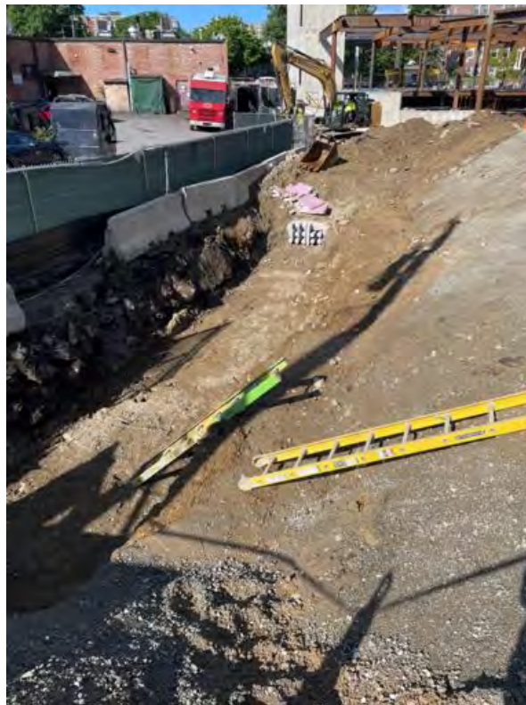
Ductbank excavation.
