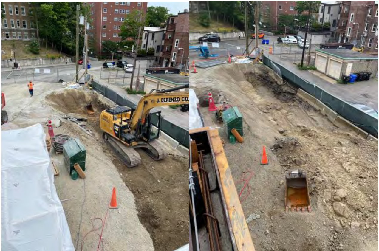
Excavation for ductbank.
