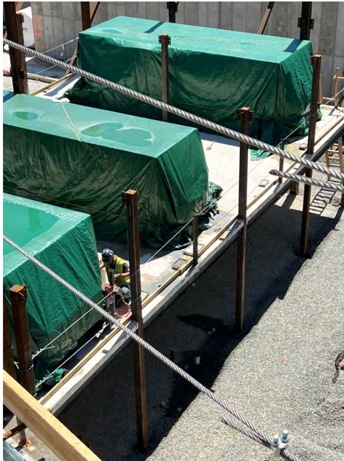
Coring for plumbing underway on mezzanine in area A
