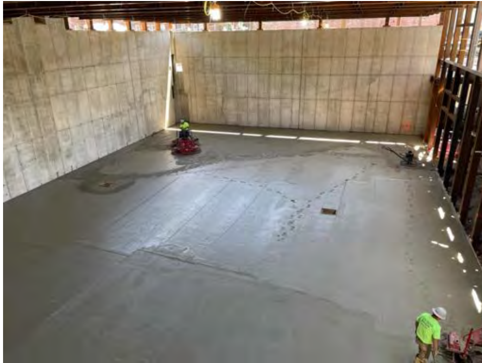
Gym slab on grade poured.
