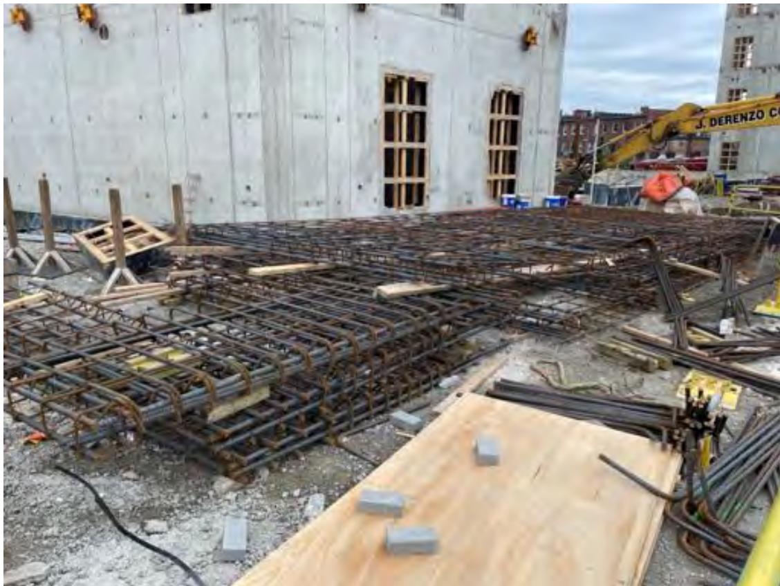
Rebar cages for Core AB.
