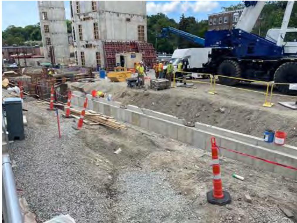
Wall stripped at BQ.
