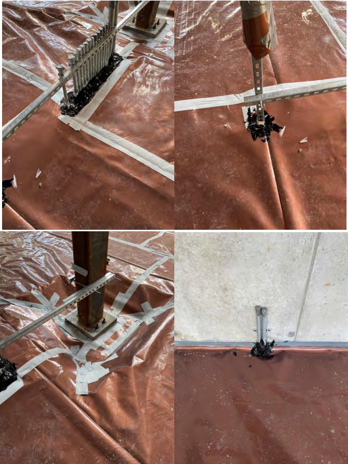
Waterproofing updates, gym slab area.
