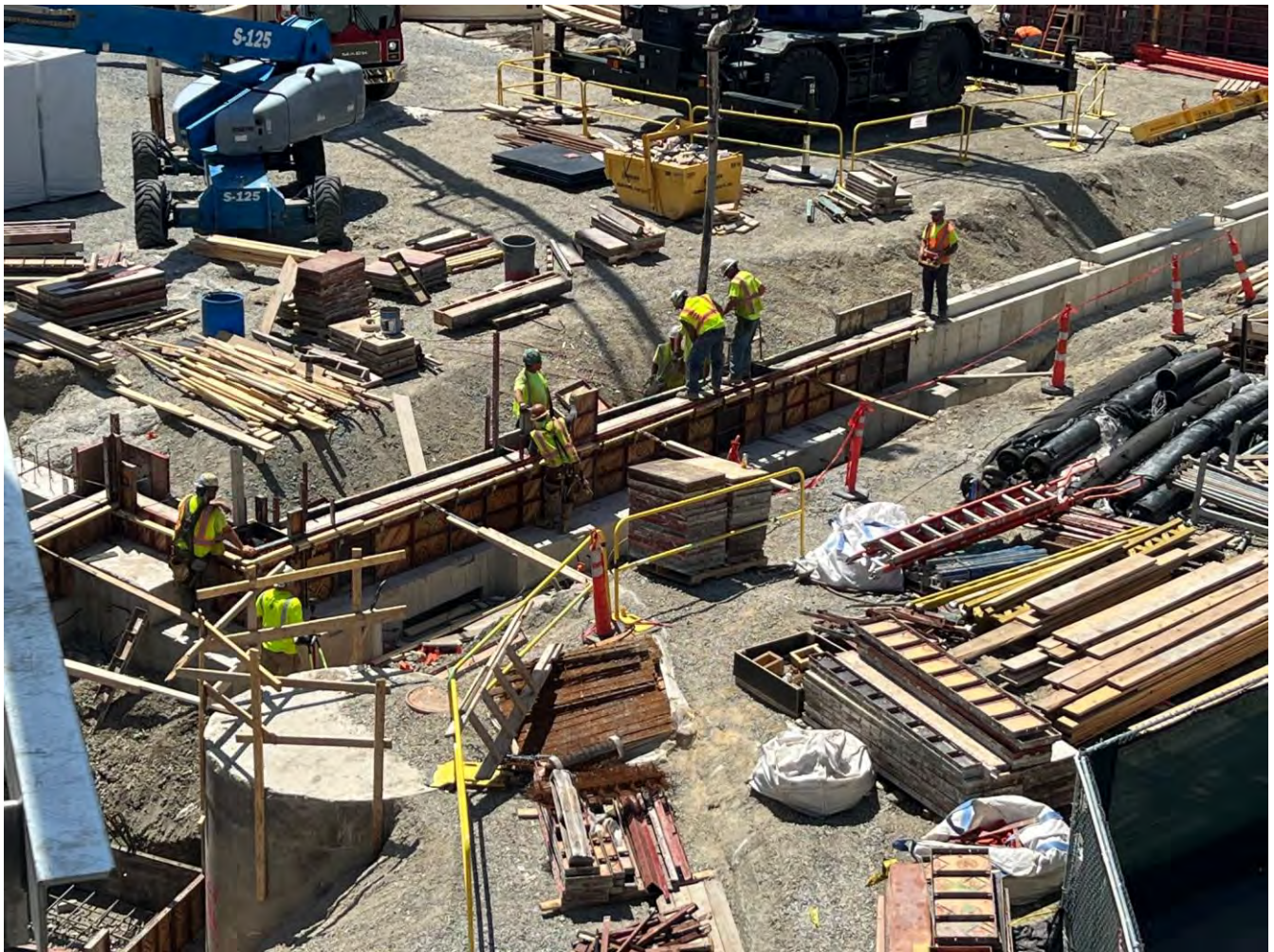
Foundation walls being poured in area B (line:B8-R1)
