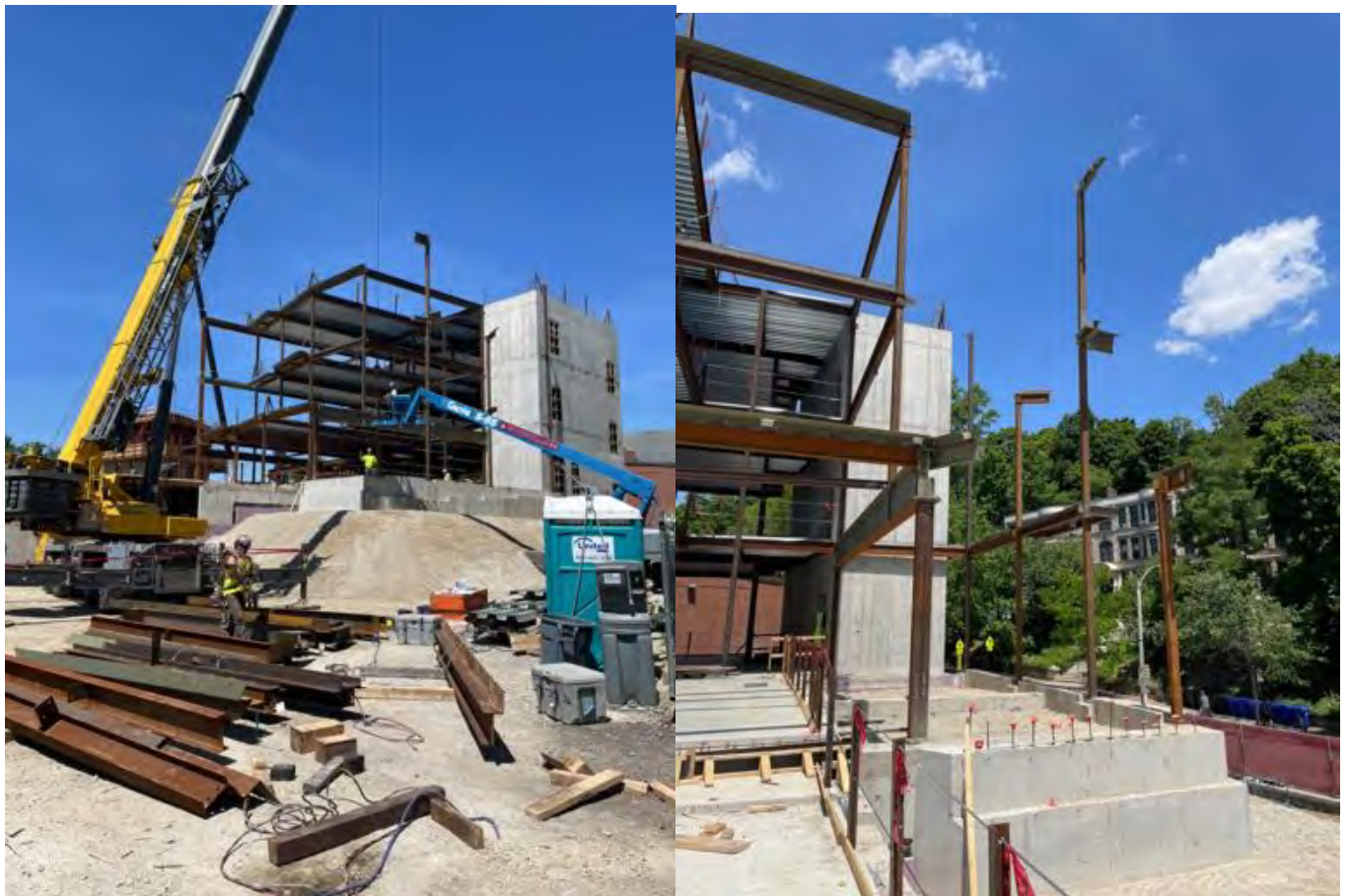
Steel erection, North side (C25).
