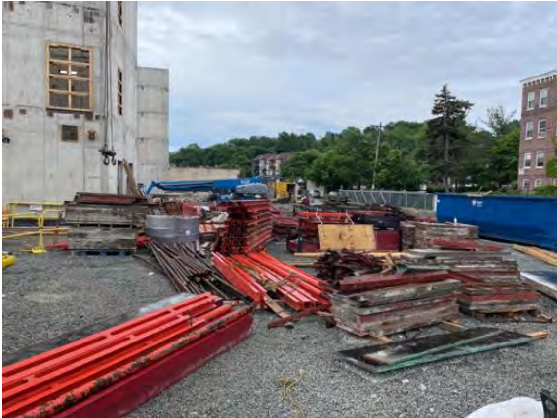
Core AB forms removed.
