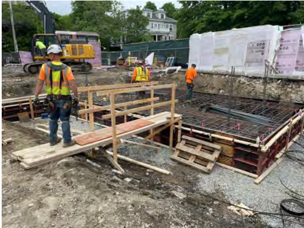
Mat slab prep, Core B.
