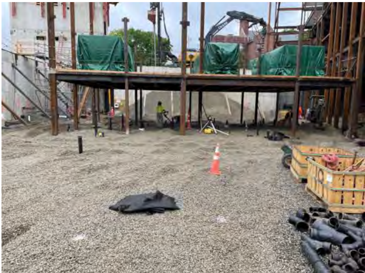
Grading crushed stone at basement level.
