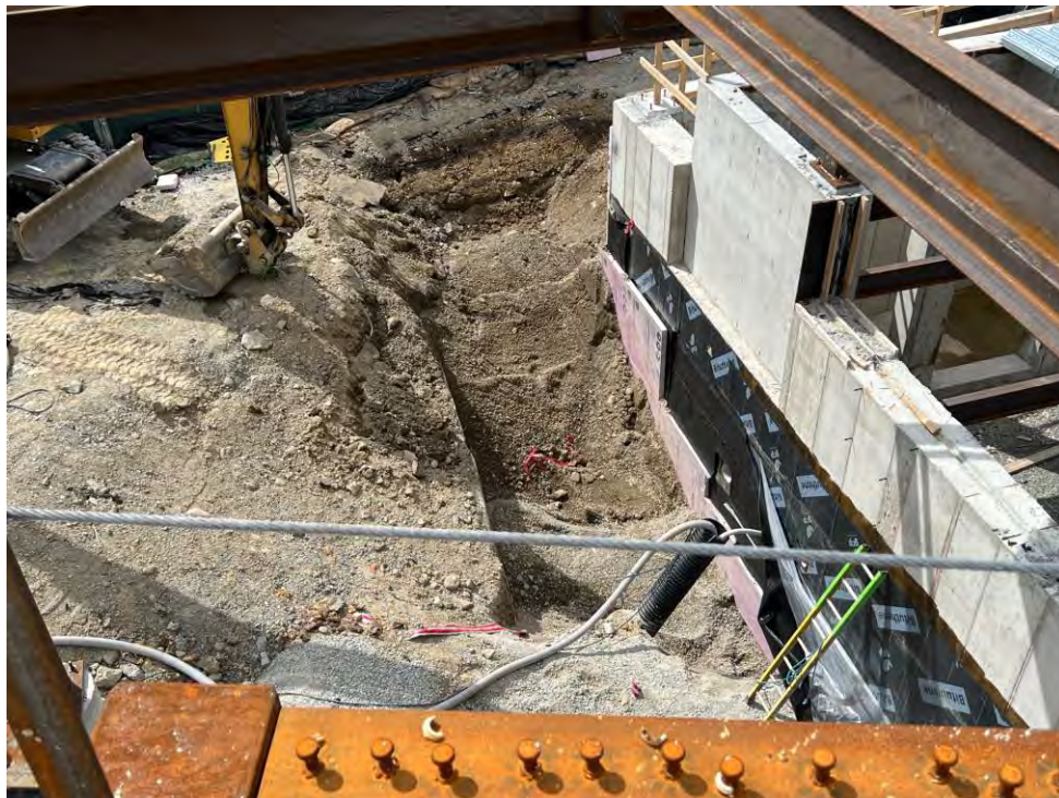
Excavation for rain leader in loading dock area (alleyway)
