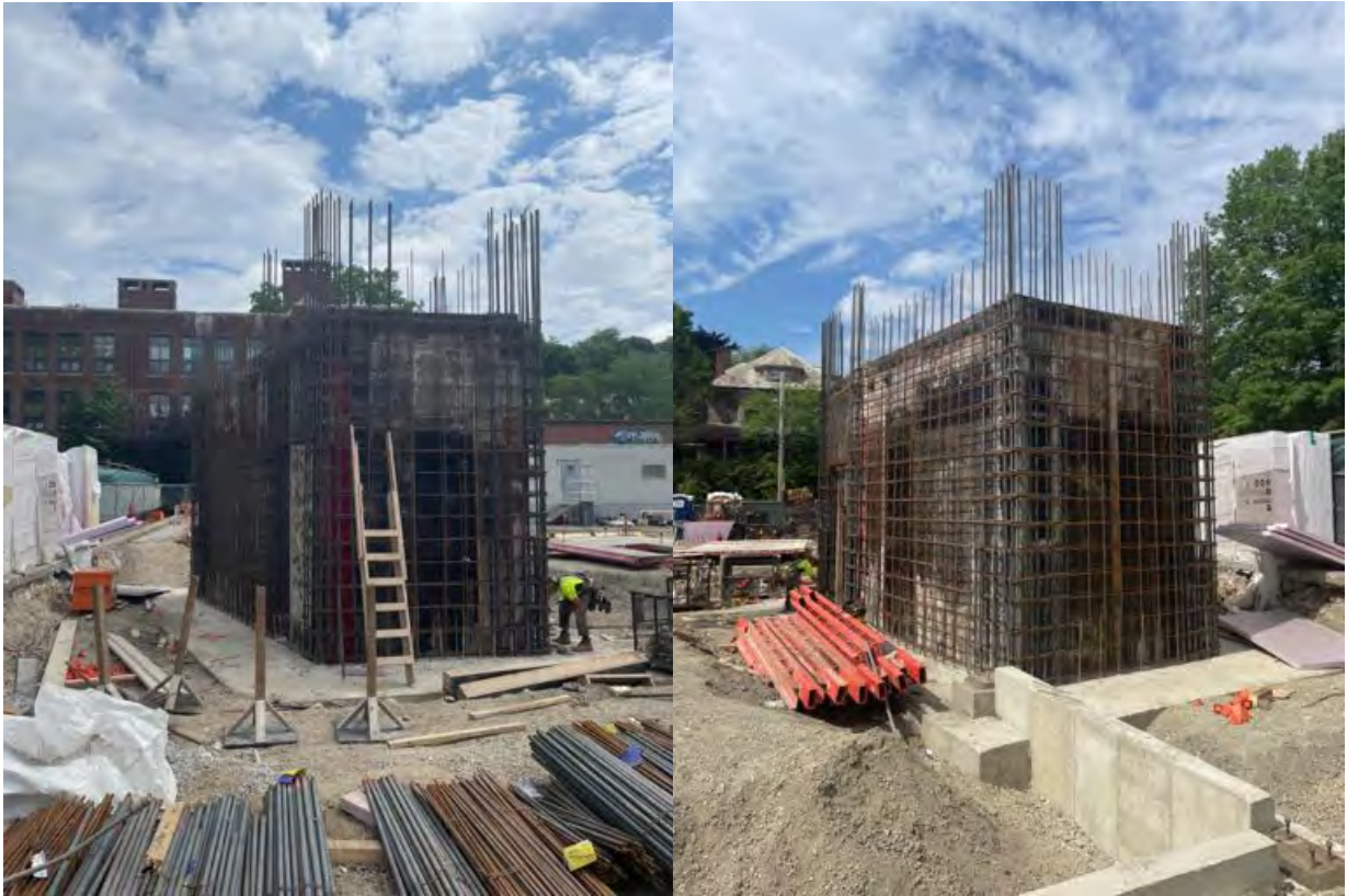
Rebar progress, Core B.
