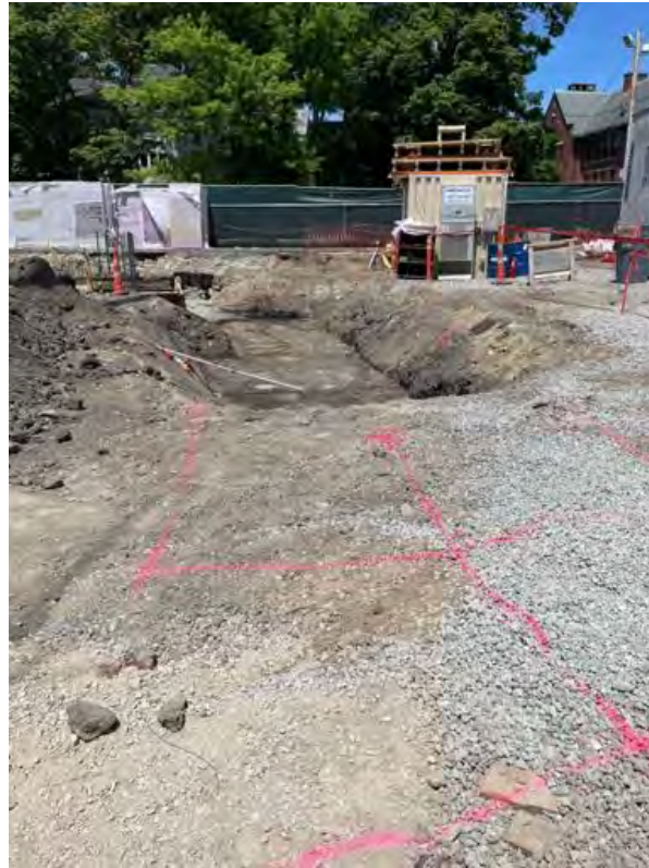
Excavation for footings, Area B.
