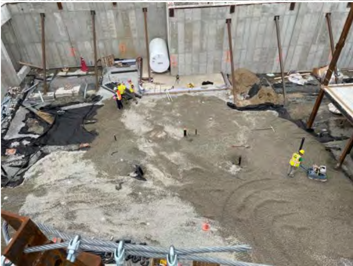
Grading basement level, areas C and A.
