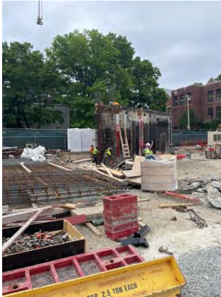
Core B rebar and forms.
