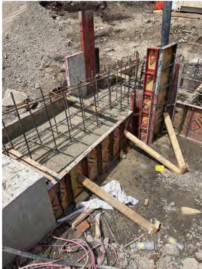
Rebar, forms and concrete at line BQ.
