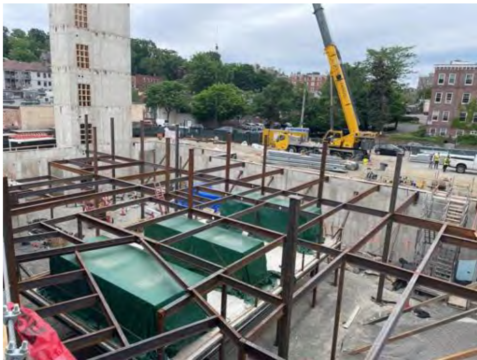
Steel erection, Area A.
