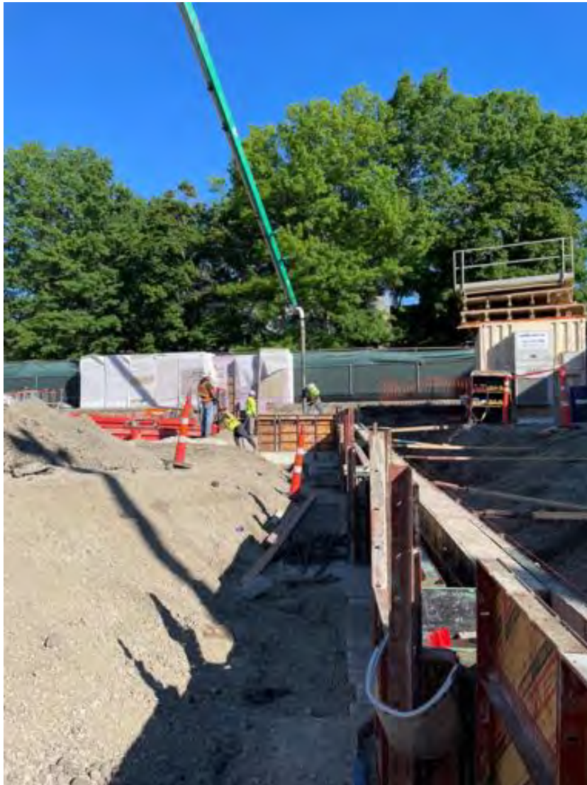
Concrete pour, walls at BQ line.
