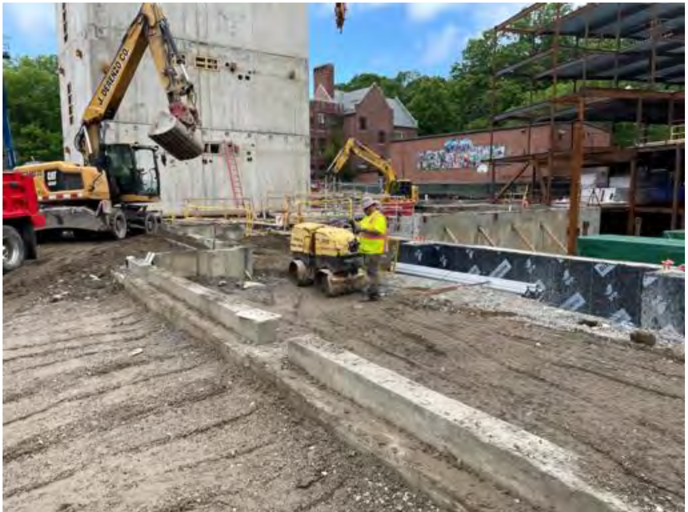
Backfill and compaction along line AD.
