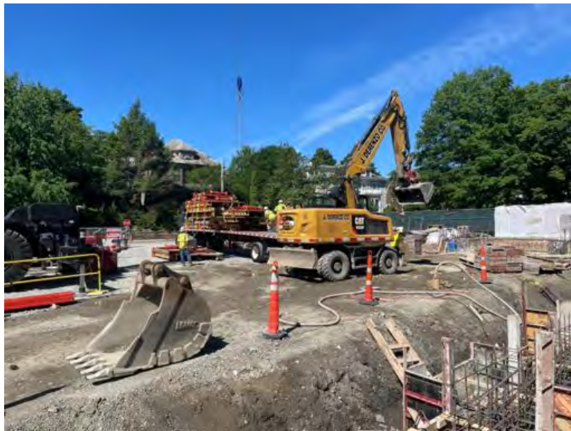
Formwork removed on truck.
