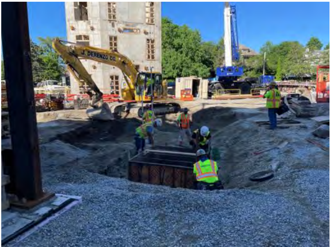
Footings adjacent to A1.
