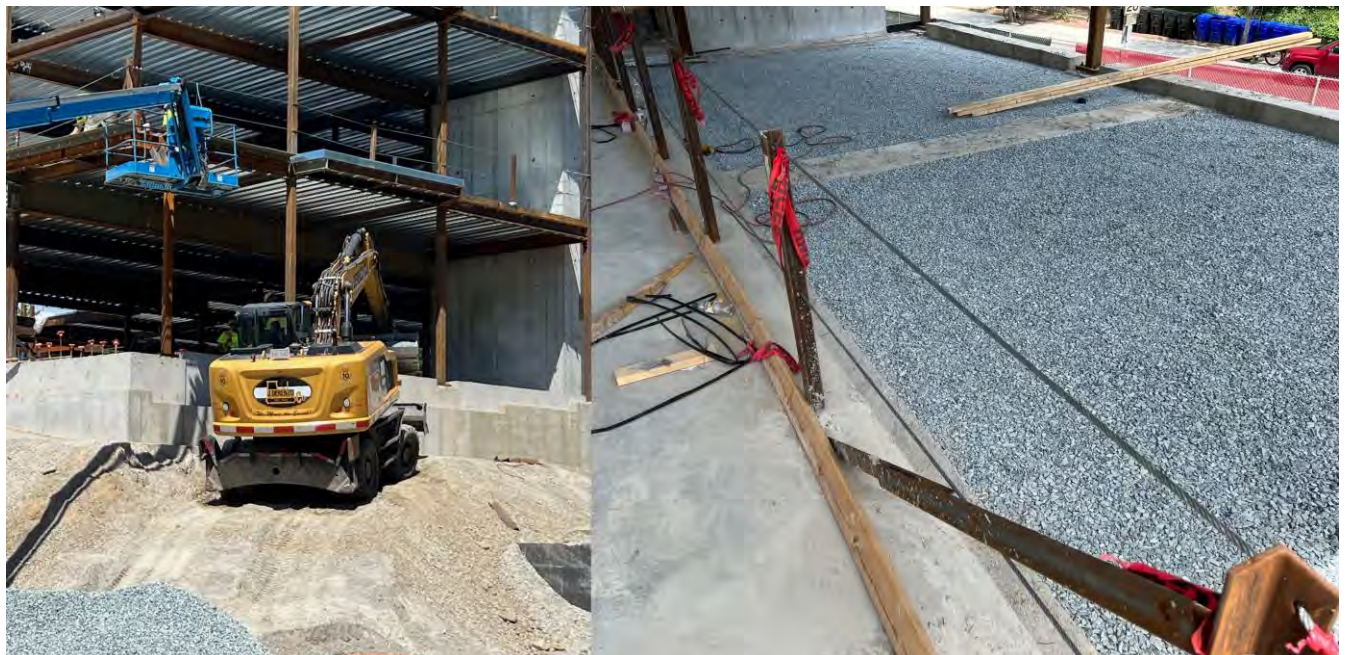
Backfill and compaction of line C25 (westbourne terrace side, Level 2).
