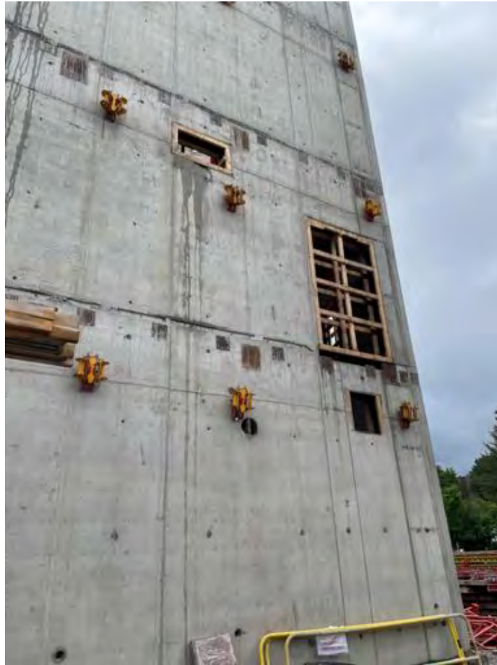
Core AB – review concrete at embeds.
