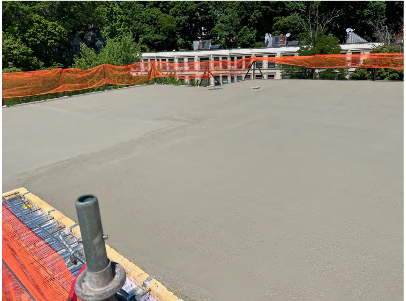
Slabs on deck being poured and finished
