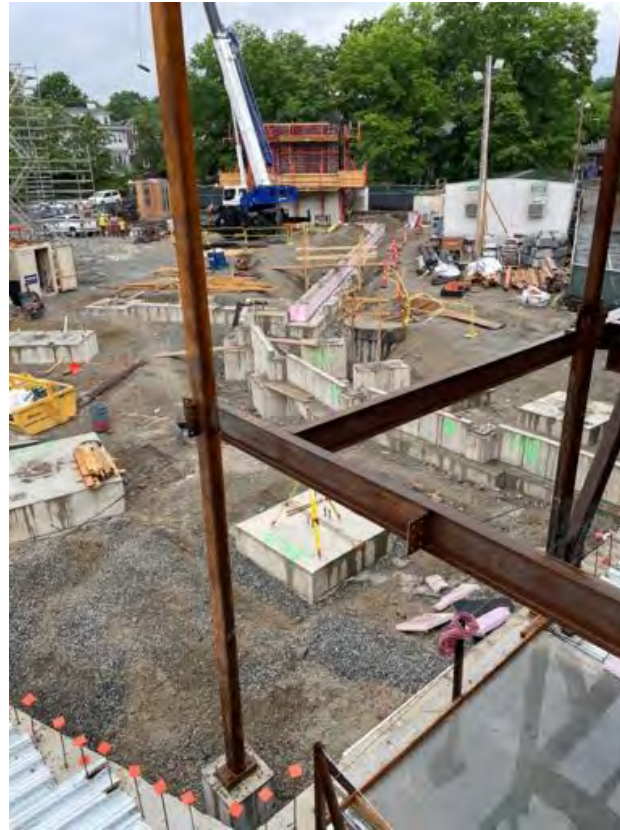
Base plates set and grouted, Area A/B/C.
