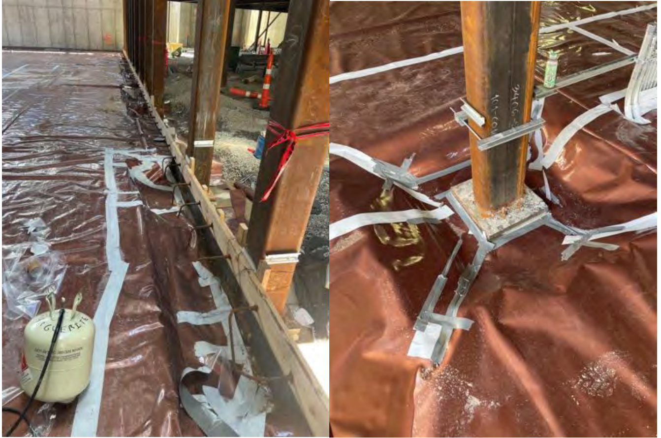
Waterproofing @ gym slab. Minor corrections to follow in Stego report.
