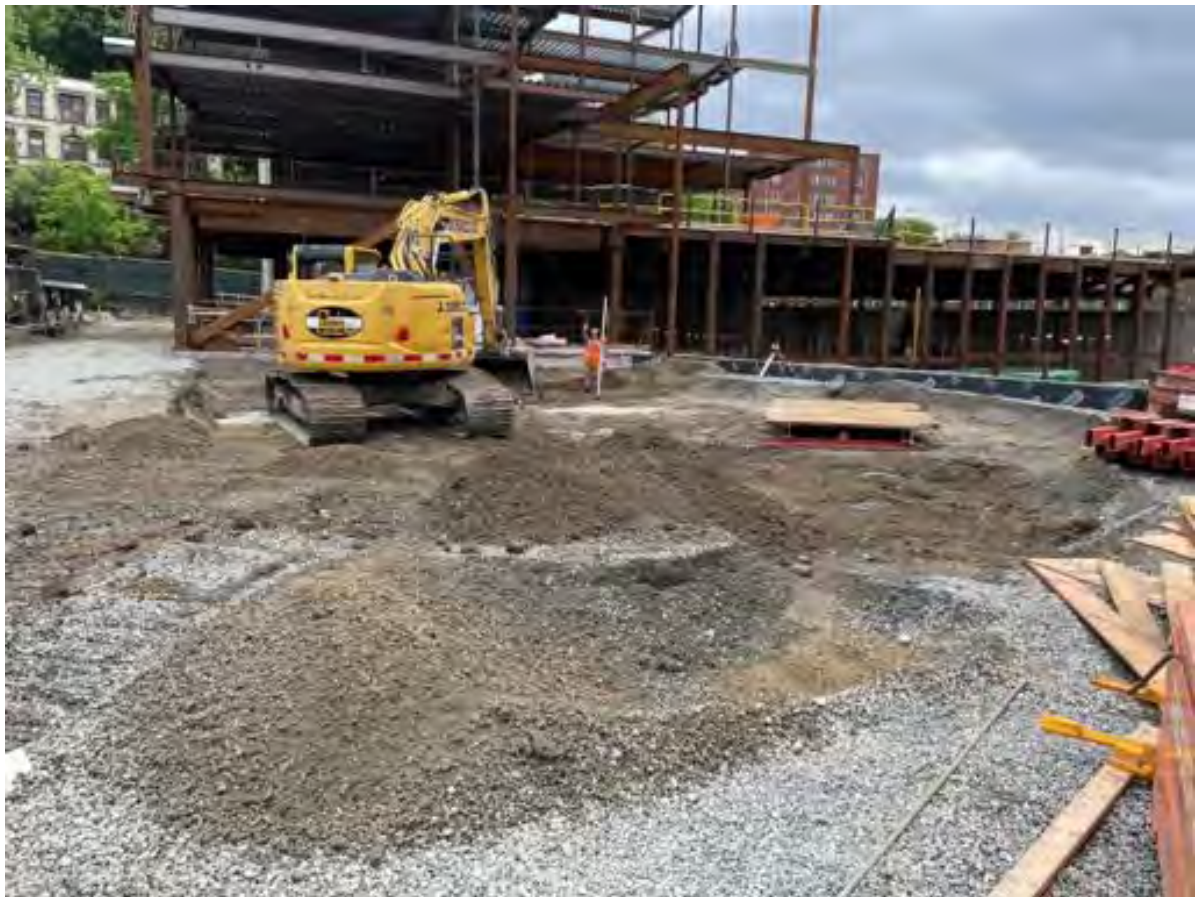
Excavation for footings adjacent to line A1
