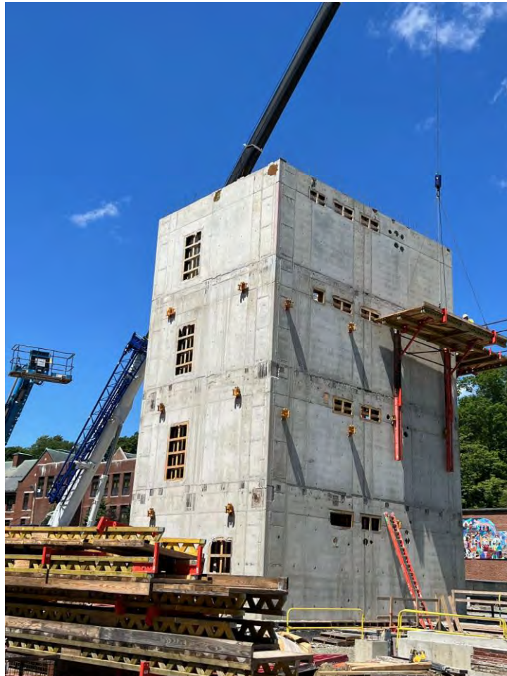
Core AB final forms being removed.
