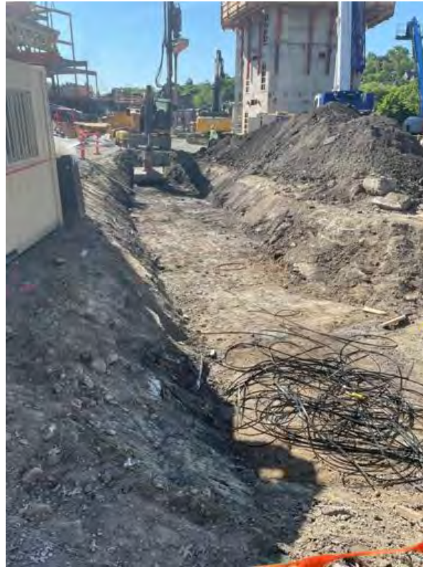
Excavation at Area B footings.
