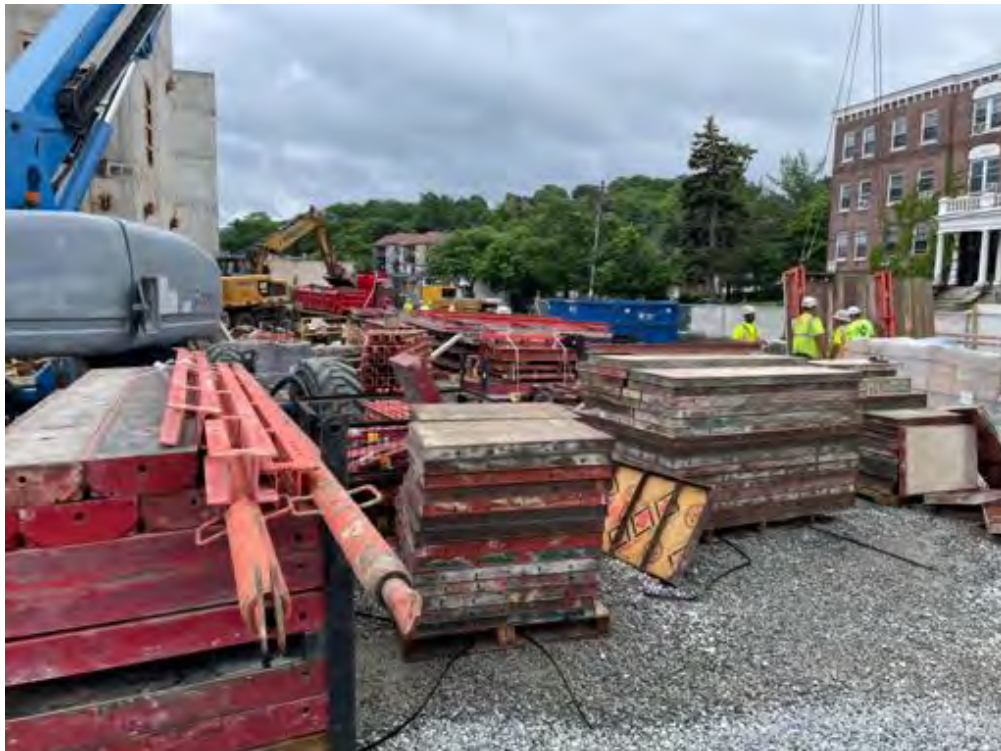
Concrete formwork from Core AB.
