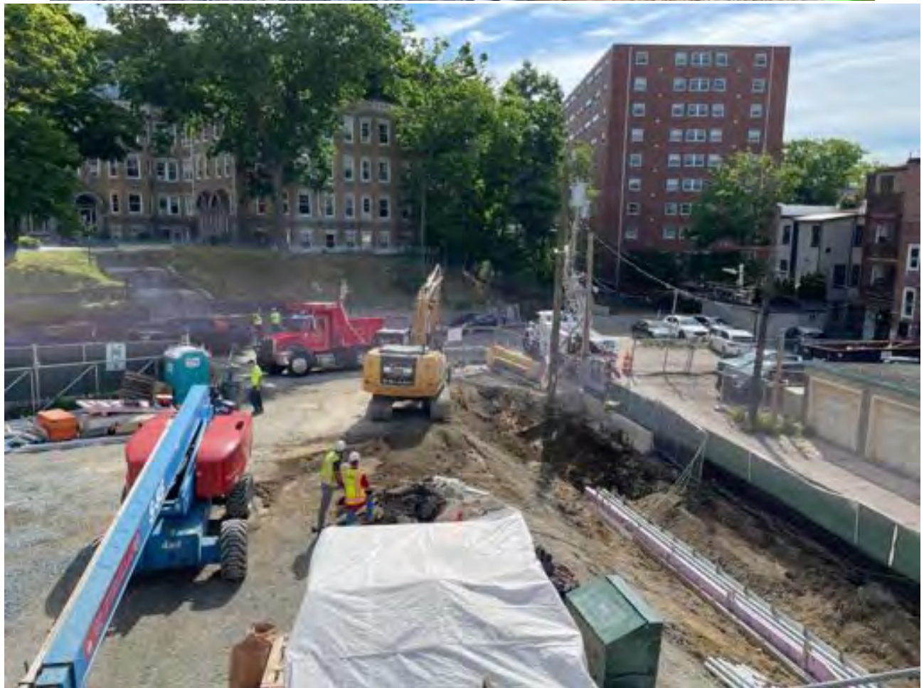
Duct bank work along alley/Westbourne Terrace. Eversource on site to stabilize pole during excavation.
