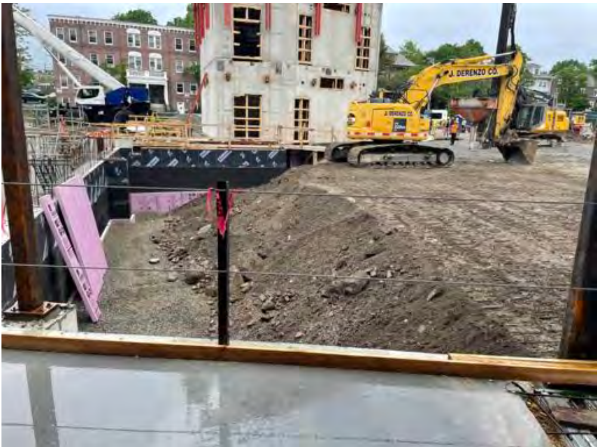
Backfill at wall A1.
