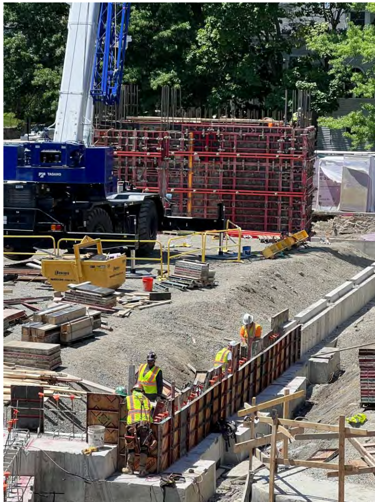
Core B level 1 forms complete. walls being formed up on line BQ.
