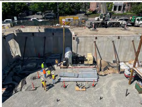
Conduit and generator crane picks.
