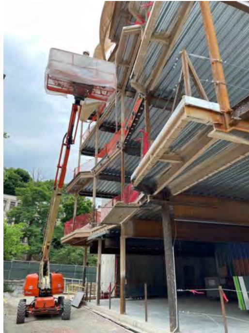
Spray Fireproofing ongoing, West and North perimeter.
