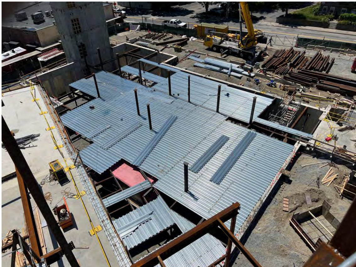
Progress installing metal deck, Area A level 1.
