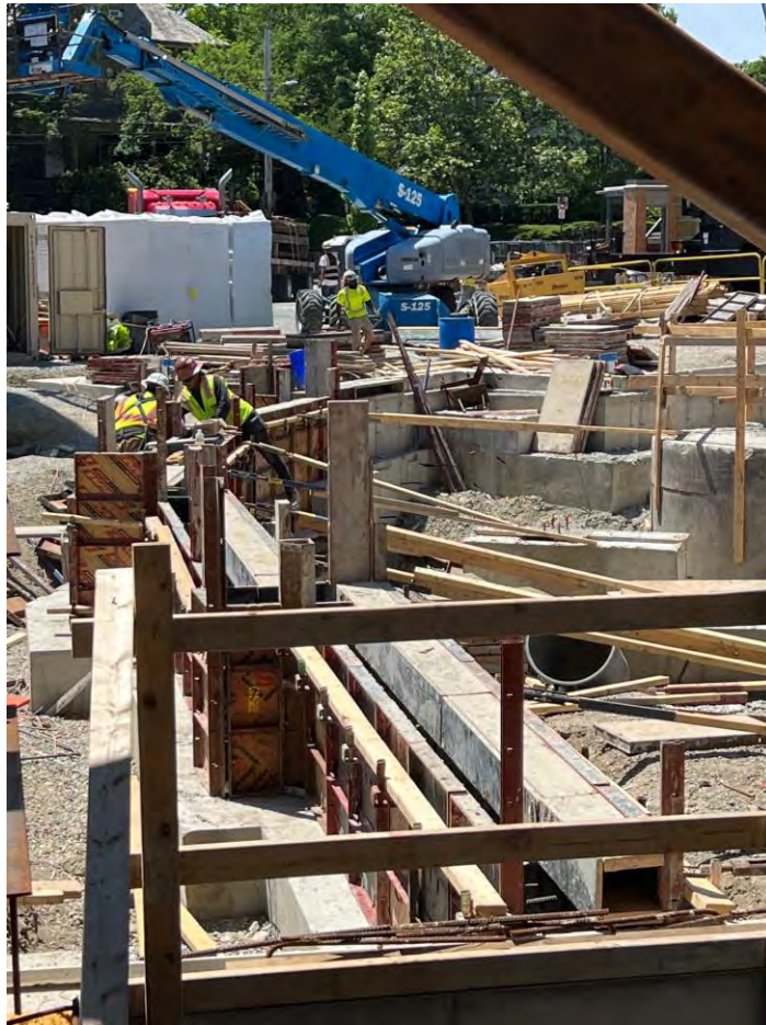
Foundation walls being formed up connection area B & area C (line:R1-C2)
