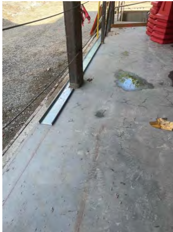
Exterior perimeter track installation started, 1 st and 2 nd floors.
