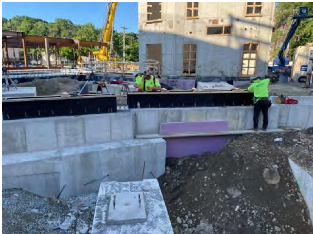
Forms installed at A/B/C.
