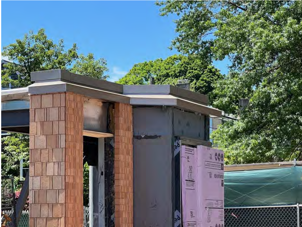
Roof edge work completed on mockup
