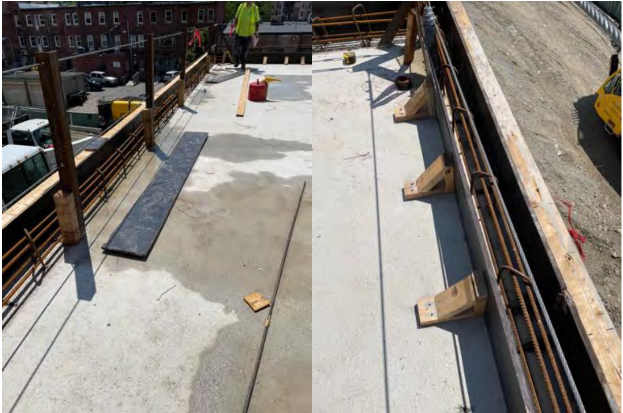
Curb forms at playground.
