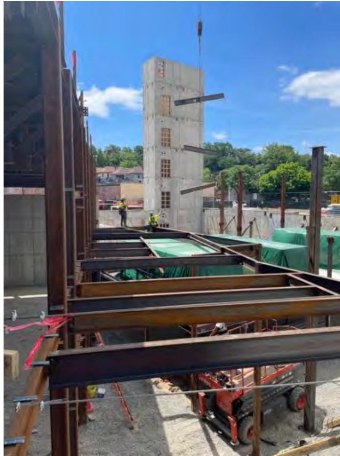
Steel erection, Area A.
