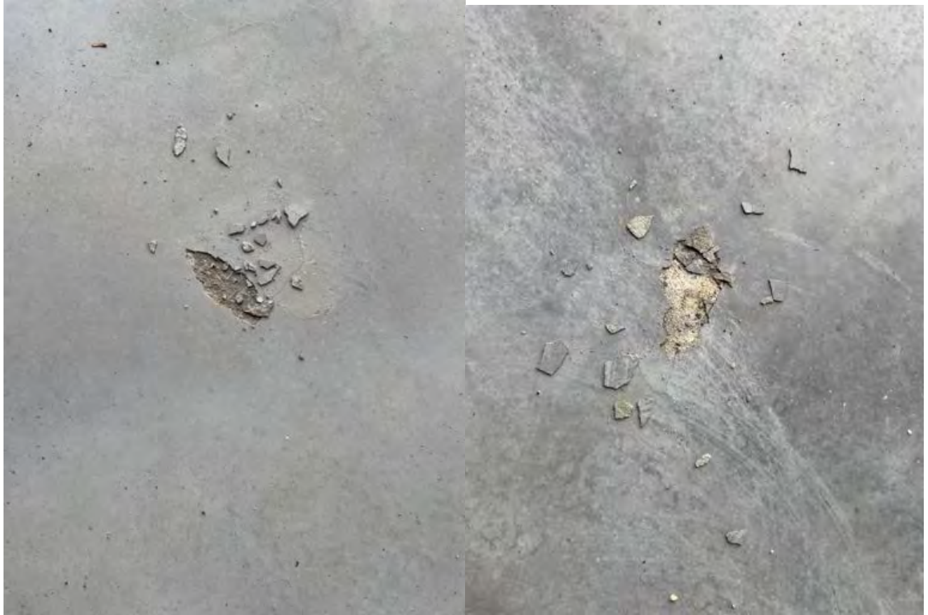
Spalling at deck C2.
