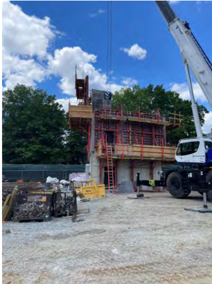
Core B – forms raised to 3 rd lift.
