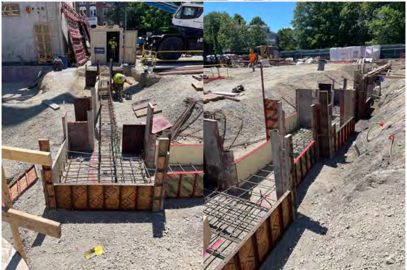
Rebar and forms, Area A/B/C.
