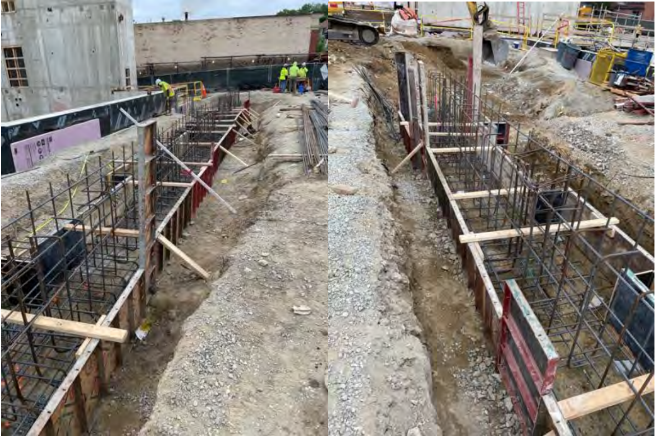
Footings at line AD.
