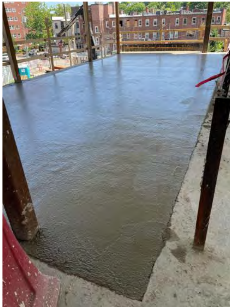
2 nd floor slab poured.
