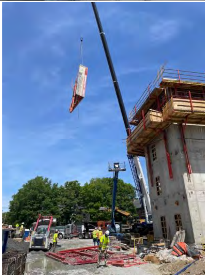
Stripping forms, Core AB and wall AD.
