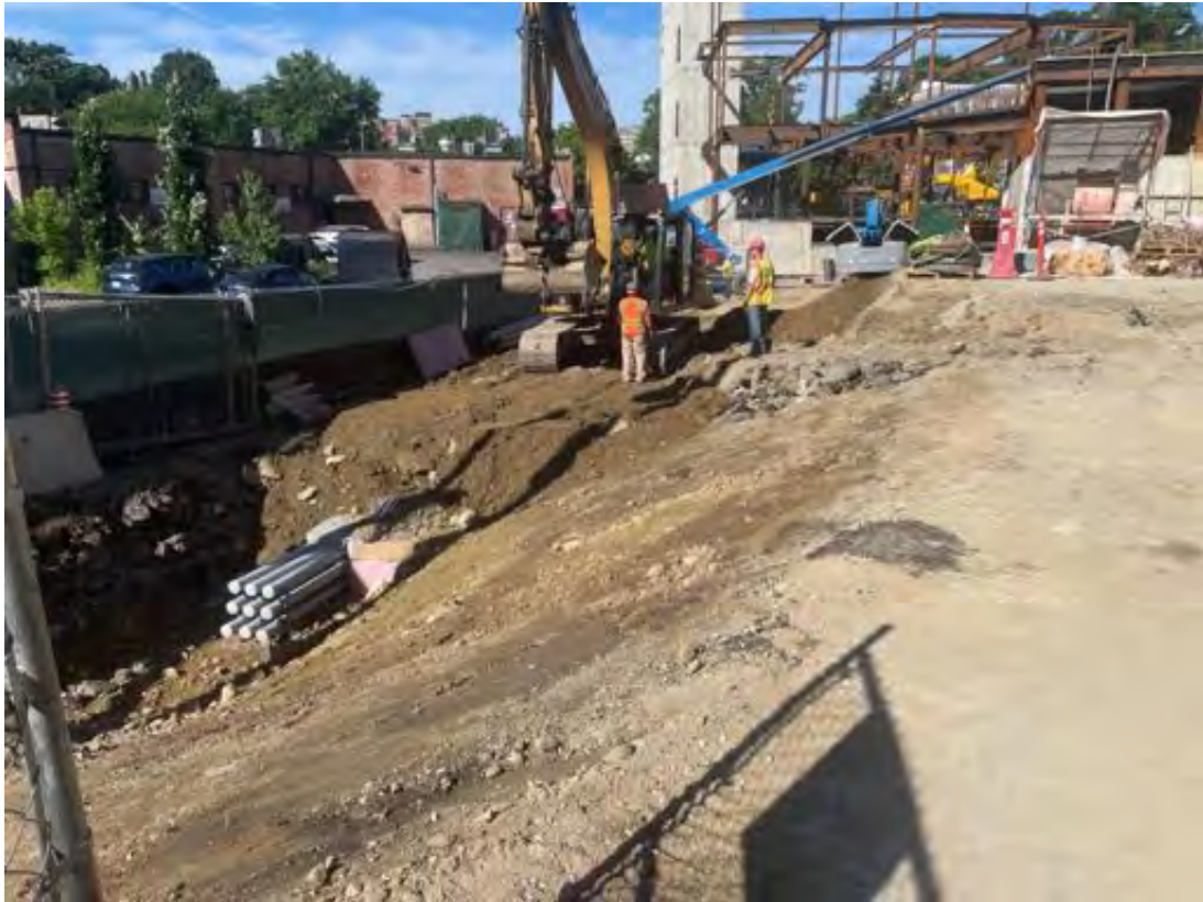
Ductbank backfilled.
