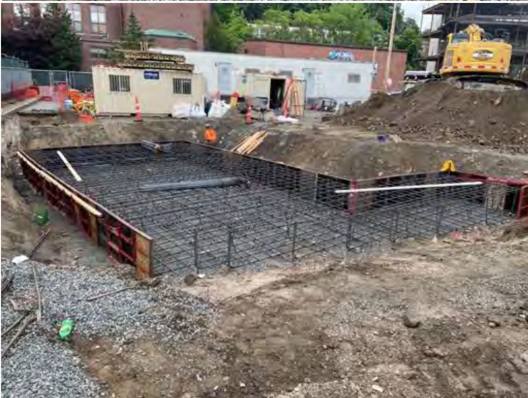
Excavation and rebar at mat slab, Core B.
