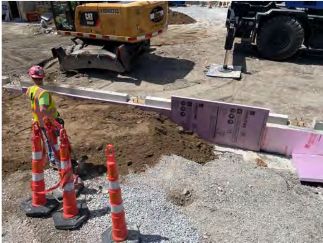
Backfill at line BQ.
