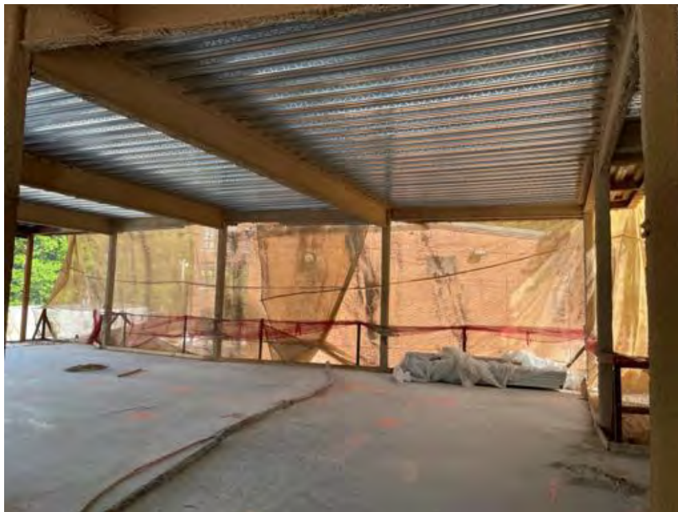
Spray fireproofing, 2 nd floor.
