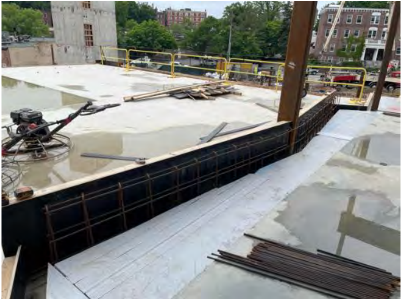
Forms, rebar and insulation at exterior edge of building.
