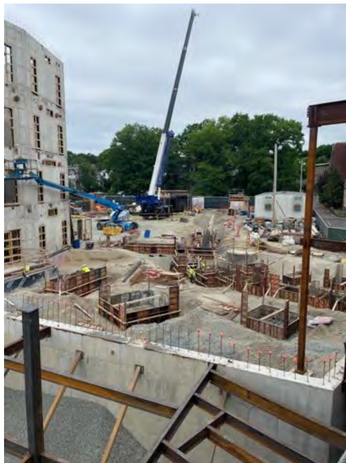
Forms and rebar.
