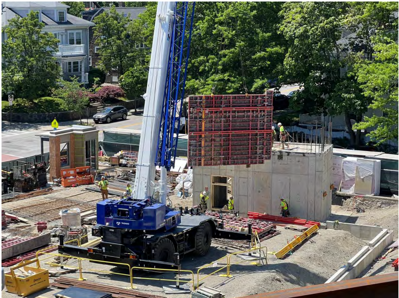
Core B level 1 – platforms installed, forms removed, and rebar cage for level 2 being built.
