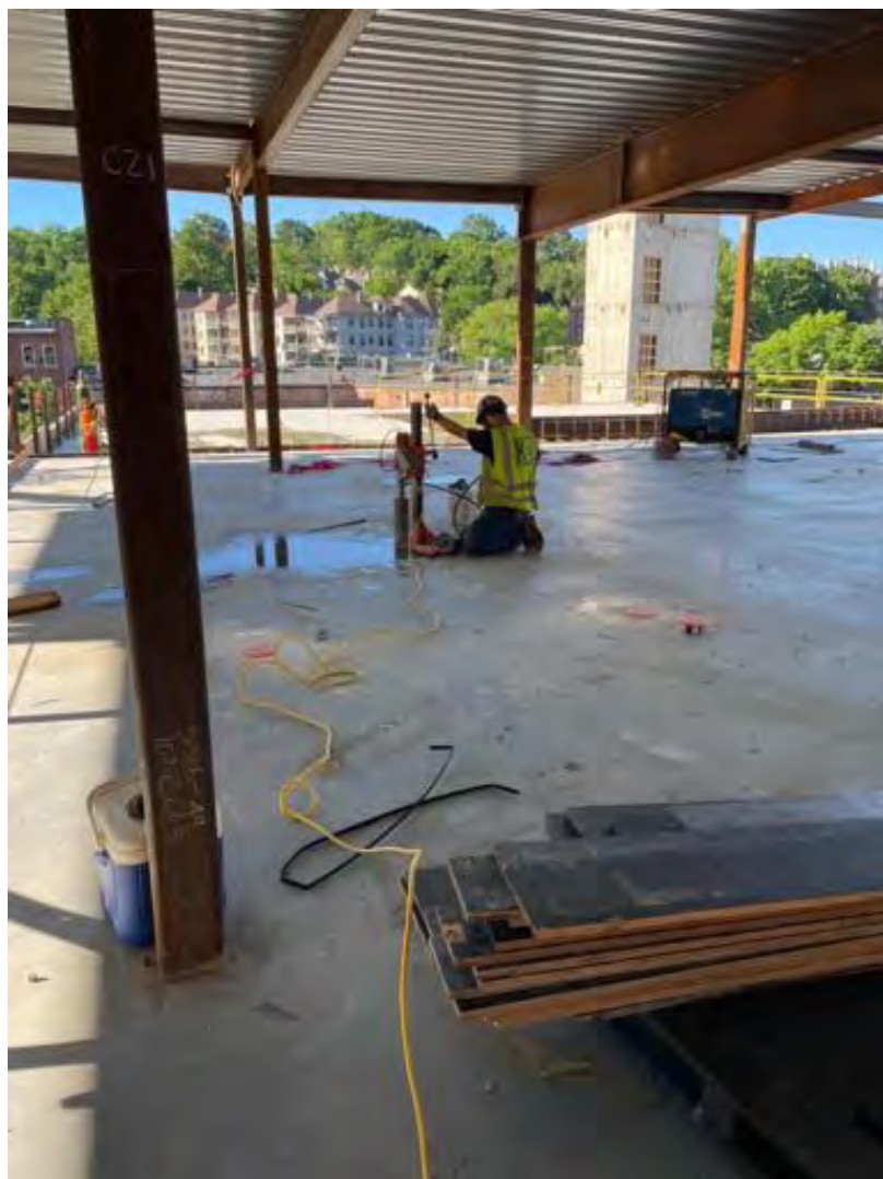
Plumbers coring on Floor 2.
