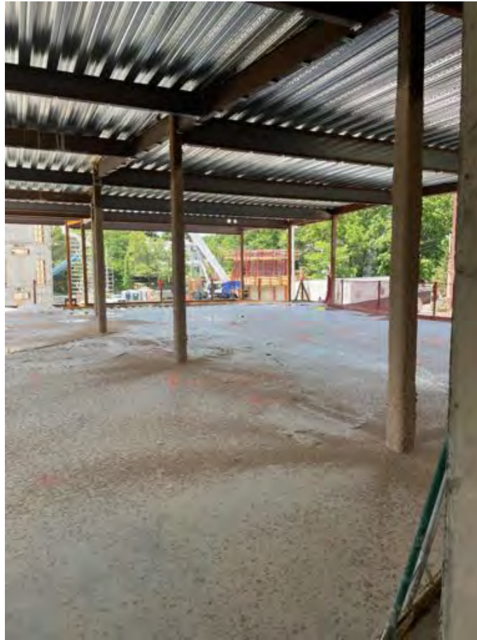
Spray fireproofing, 2 nd floor.
