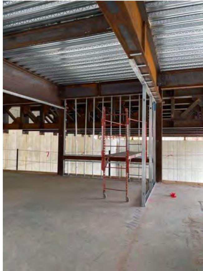
Light gauge metal framing, C1.
