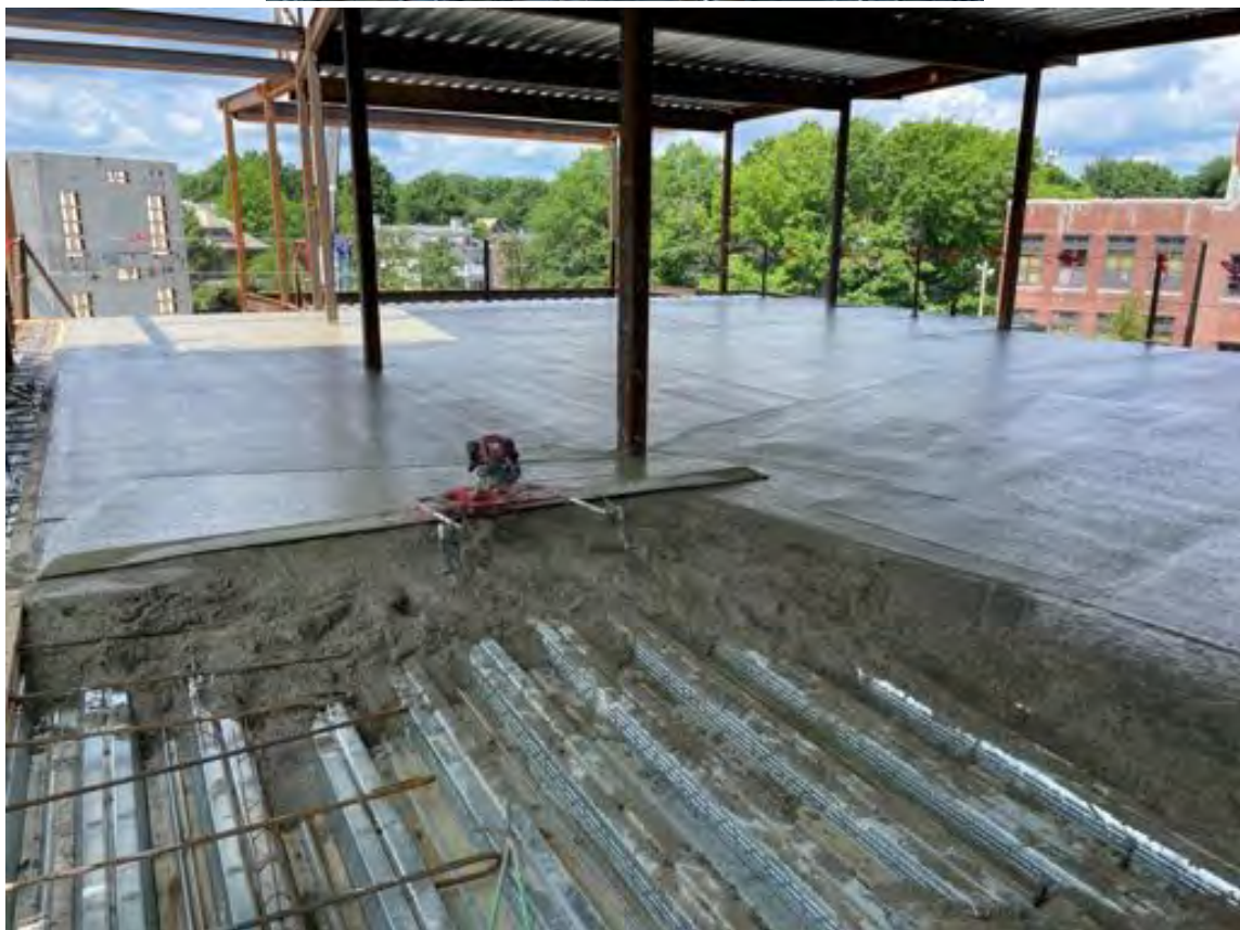
Concrete pour, levels 3 and 4.
