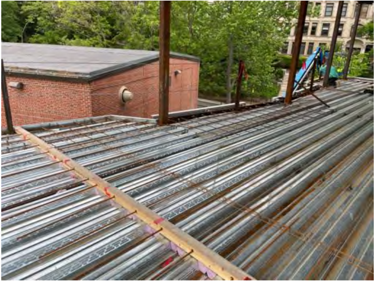
Rebar and bulkhead at deck C3.
