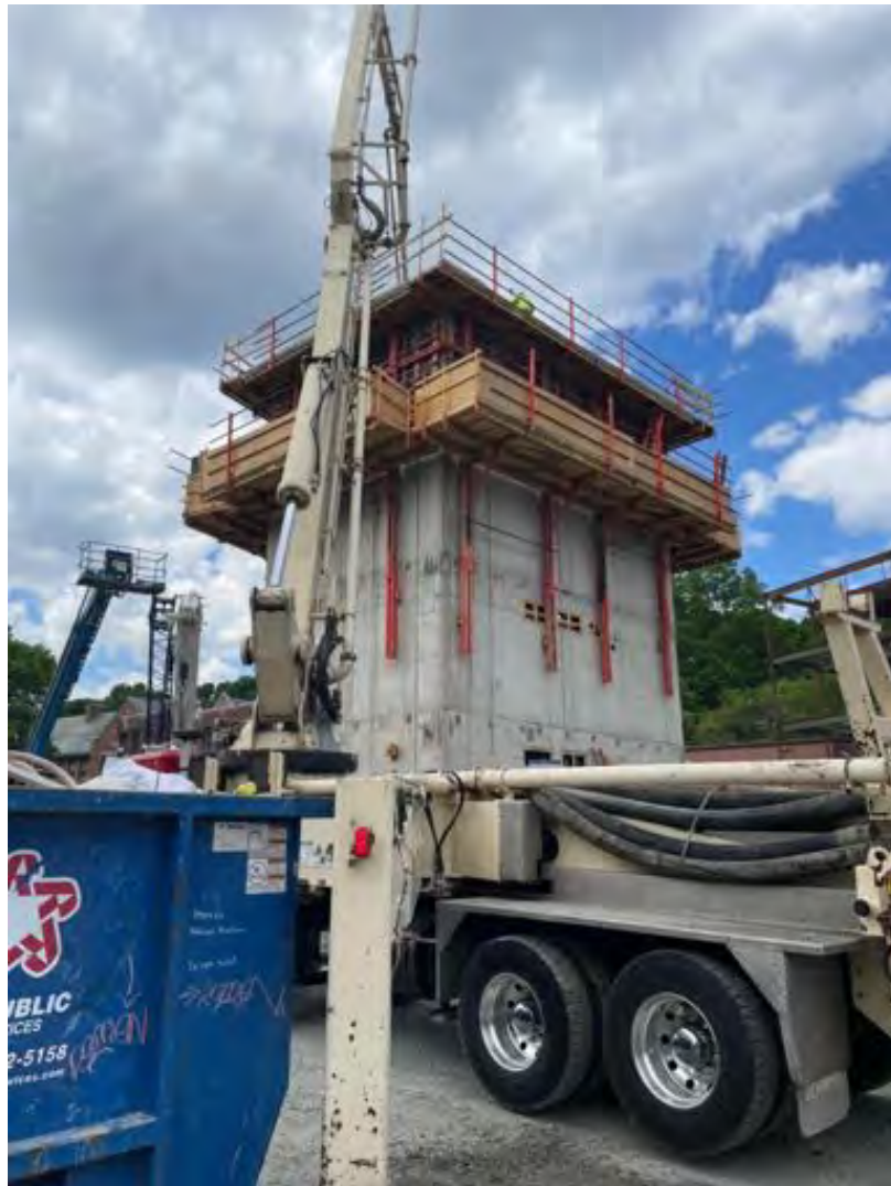
Concrete pour, Core AB and wall AD.
