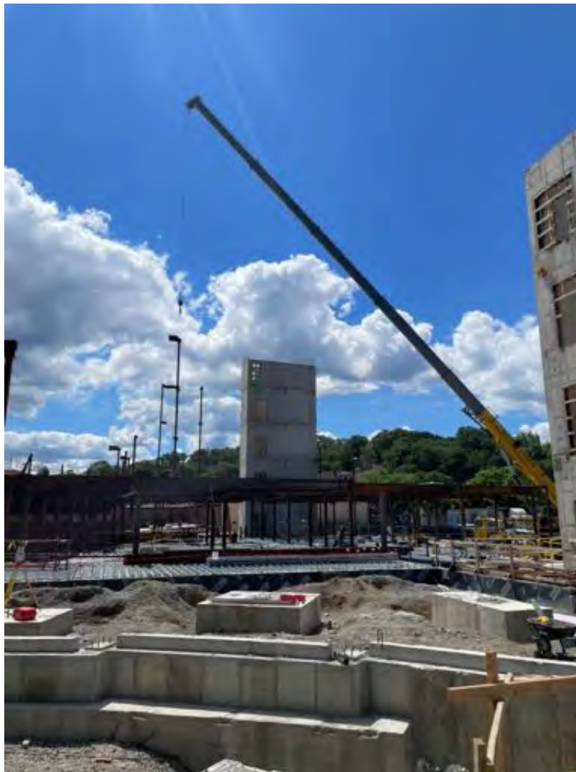
Steel erection, Area A.
