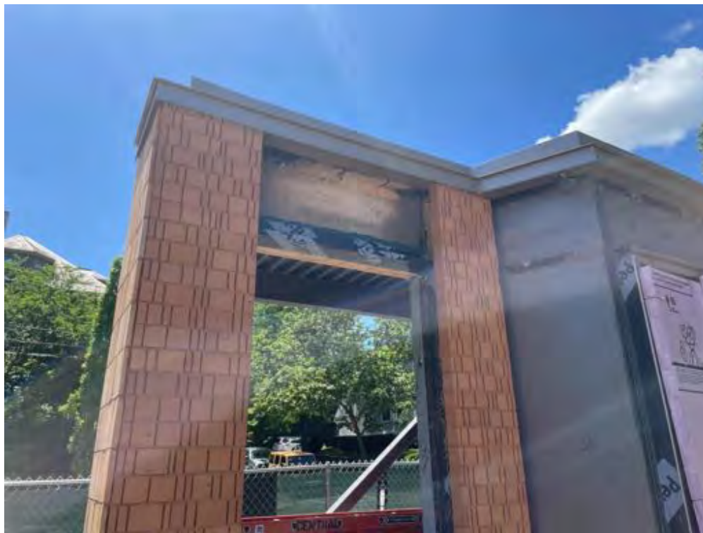
Mockup – waterproofing at window head redone.
