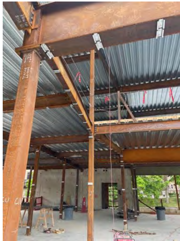
Clips installed Area C.
