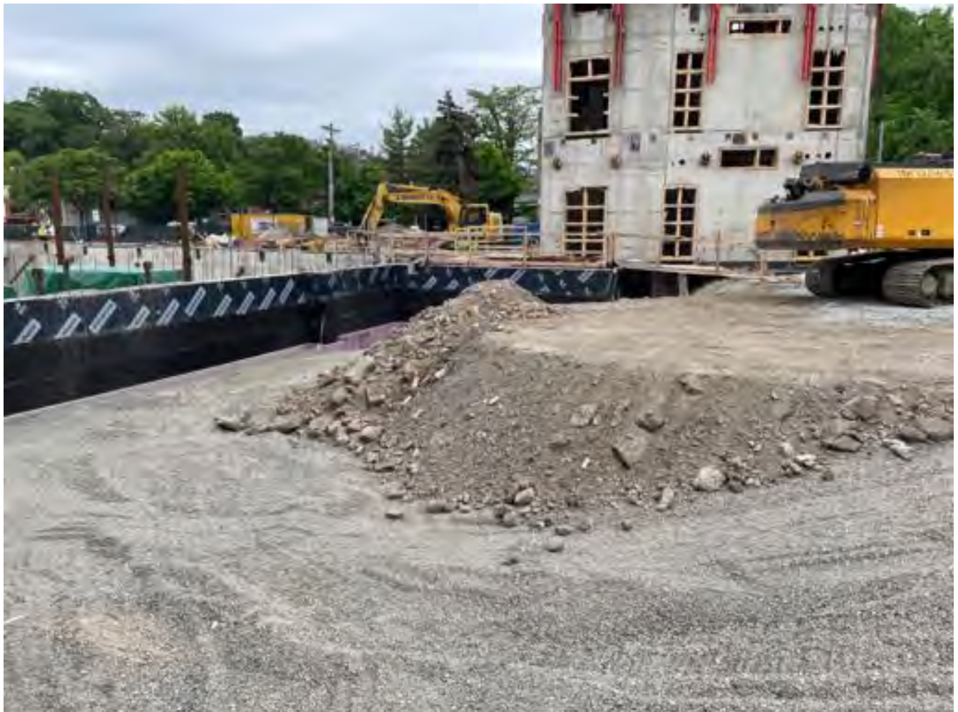
Backfill at former ramp area.
