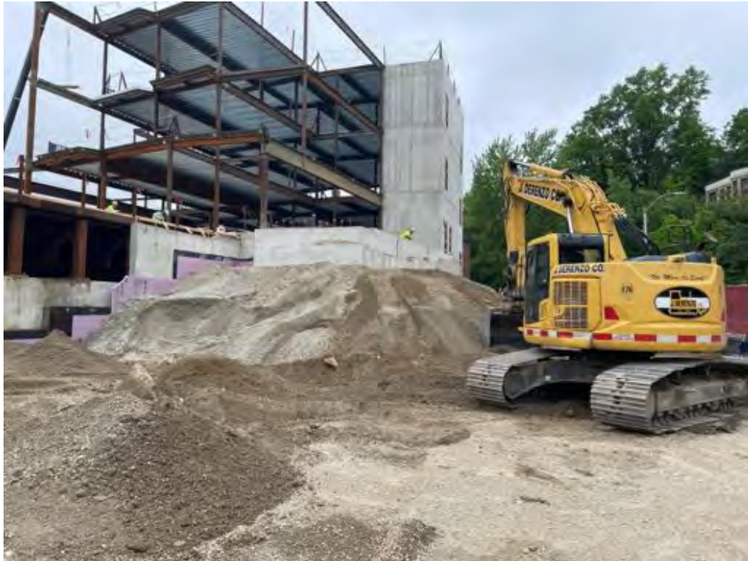
North side prepared for crane.
