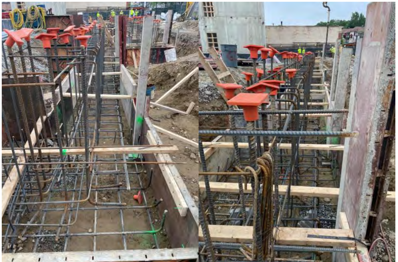
Forms and rebar, line AD.
