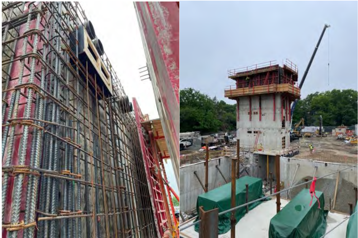
Rebar at Core AB, forms closed.
