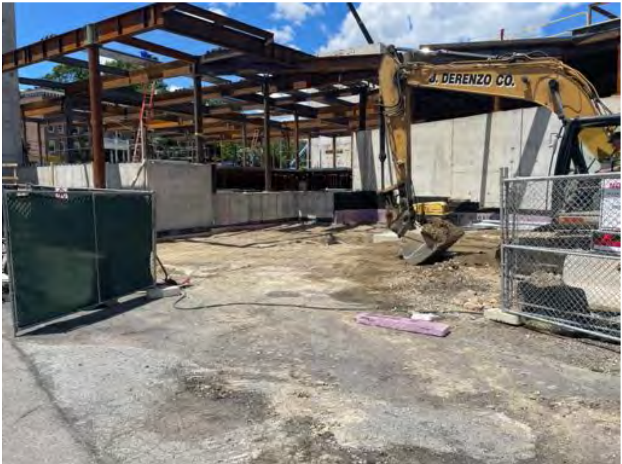
Loading dock area backfilled.
